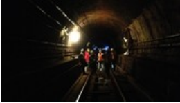
Subway Tunnel to Close
